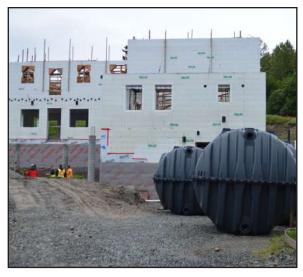
gallons of rainwater via a downspout. The rain collected will be used for a variety of basic home and landscape needs, including irrigation, vehicle washing, flushing toilets, and running laundry. Similar projects under the Net Zero Energy initiative are expected to take place in the near future for approximately 20 other homes across Canada.
