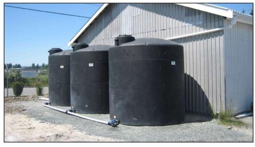
AW 9,000 USG system comprised of 3 tanks that collects from 5000 sq. ft. roof and supplies water for filling mobile equipment and washing equipment.
