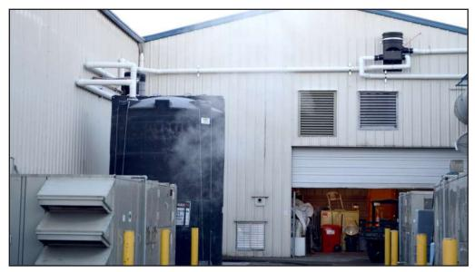
We worked with Abbotsford Water & Sewer Services to create an 8,000 USG ASTM rated poly tank with engineered seismic tie-downs. This custom ranwater systems collects from 48,000 sq. ft. of roof area to collect up to 1.6 million US gallons per year to flush over 30 bathroom fixtures. It was designed to meet the demands of a tradeshow day which can commonly use up to 8,000 US gallons.
